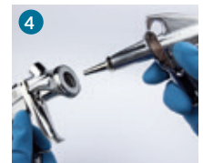
4 Dry paint passages by using a blow gun
