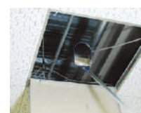
For inspection in ceiling
